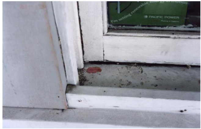
A D-I-Y test can be performed in seconds with a Lead Check Kit. If the swab turns pink, lead is present.
